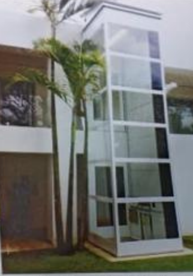
Glass Protected Structure
